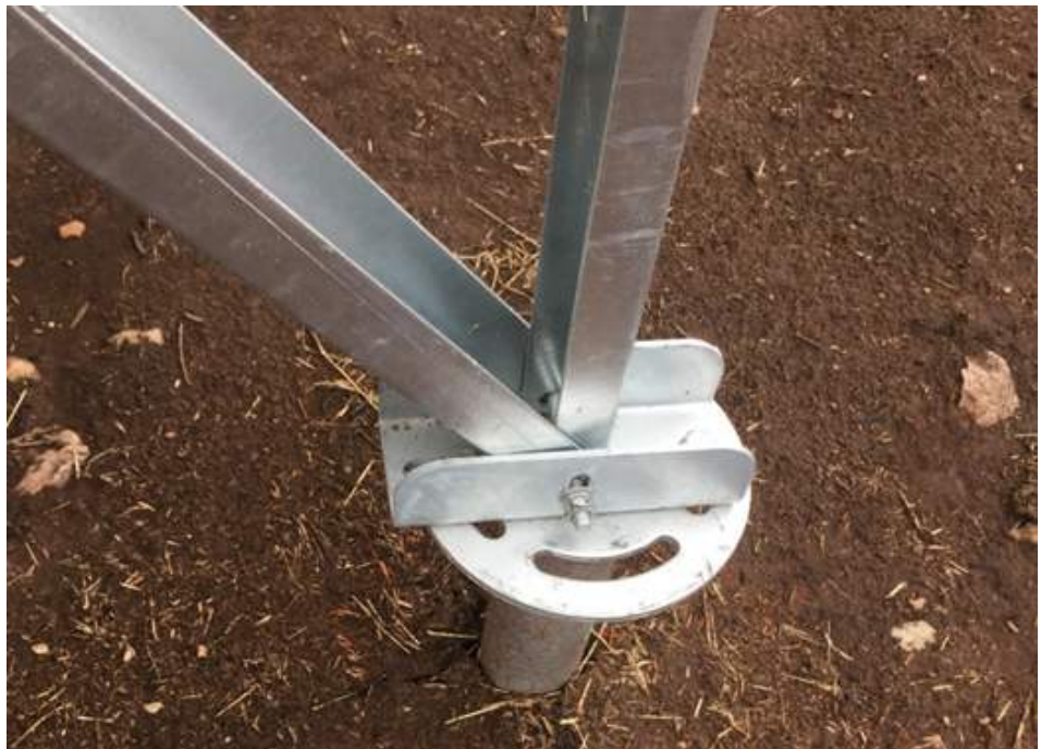
FIGURE 4-3: EXAMPLE OF GROUND-MOUNTING ARRANGEMENT (PROVIDED BY PITT & SHERRY)
