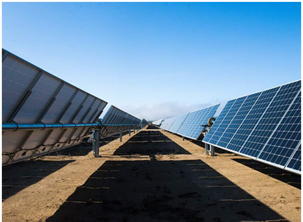
FIGURE 4-2: EXAMPLE OF PV PANELS IN SINGLE AXIS TRACKING SYSTEM (PROVIDED BY PITT & SHERRY)
