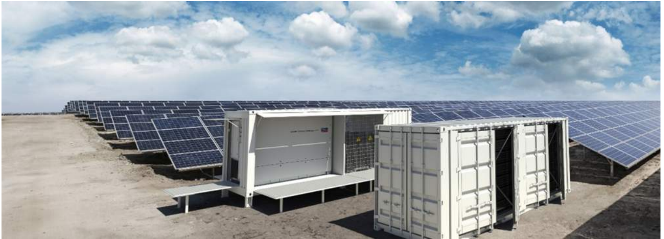
FIGURE 4-4: EXAMPLE OF PV SOLAR INVERTER & INVERTER STATION (PROVIDED BY PITT & SHERRY)
