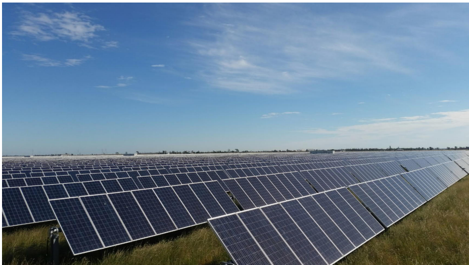
Image of single-axis tracking technology installed at Moree Solar Farm (56MW) NSW
