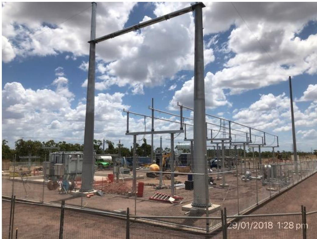
Figure 9 Electrical switchgear being installed at Wirsol's Whitsundays Solar Farm
