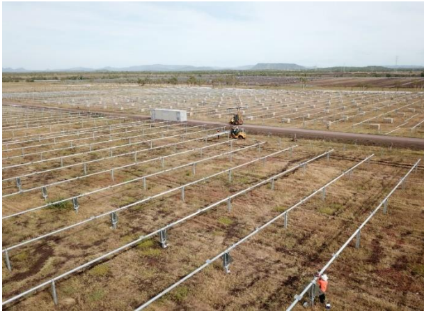
Figure 4 Pile driven steel posts with tracker assemblies
