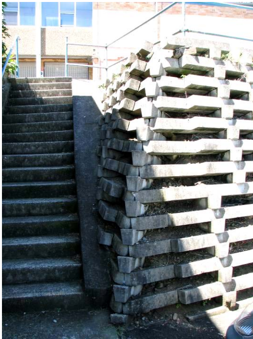
Crib wall supporting western side of car park lining western side of service wing.
