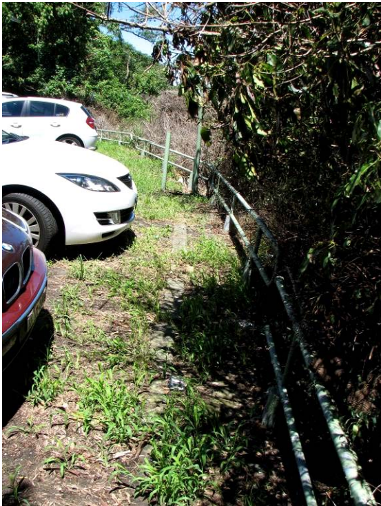
Leaning fence at crest of fill batter to west of main hospital wing.
