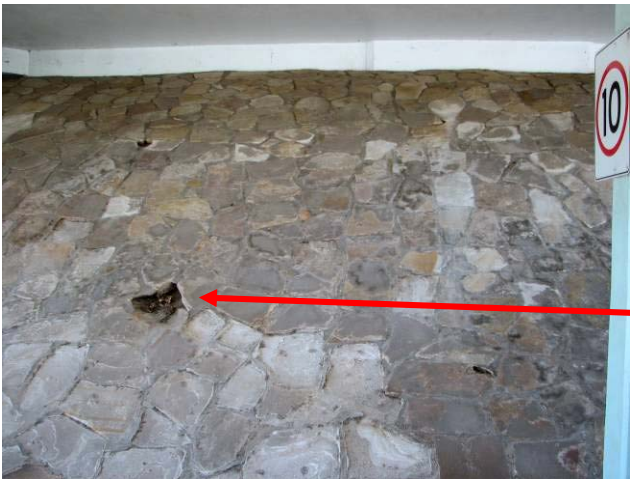
Sloping faced sandstone masonry wall below central portion of main hospital wing.
