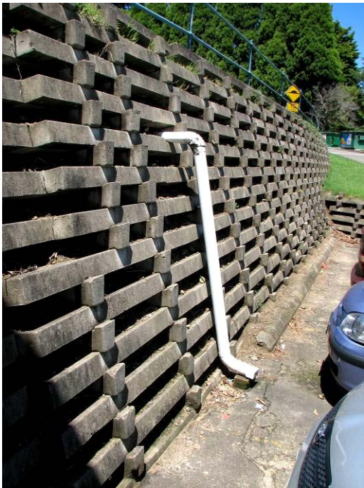
Crib wall supporting western side of car park lining western side of service wing.
