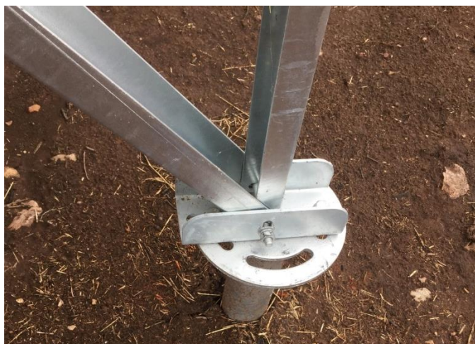
Figure 2-5 Example ground mounting arrangements
