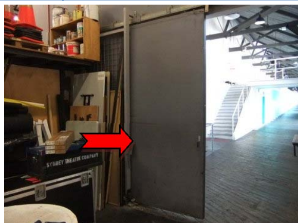
Photo 6. Level 3, interior, workshop entrance, SMF-containing fire door core
