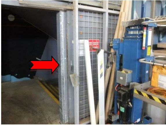
Photo 7. Level 3, interior, fire tunnel, SMF-containing fire door core
