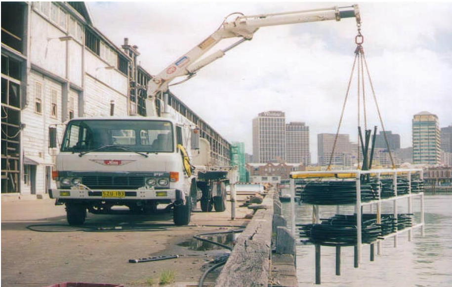
Figure 7: Photograph taken during installation of closed loop geoexchange system at Woolloomoolloo Wharves, Sydney Harbour (Source: GEOEXCHANGE Australia)
