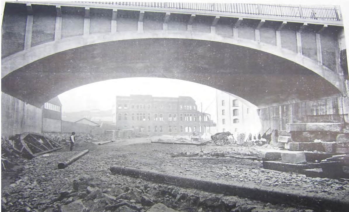
Figure 12: View west along Hickson Road showing the new bridge that spanned what was described as “deep rock cutting” through Millers Point. Wharf 8/9 is in the background and in the foreground can be seen some of the sandstone that has been extracted as dimension stone (Source: SHT Annual Report 1913 )
