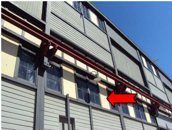
Photo 3. Exterior/interior, throughout, infill panels – suspected asbestos-containing fibre cement sheeting
