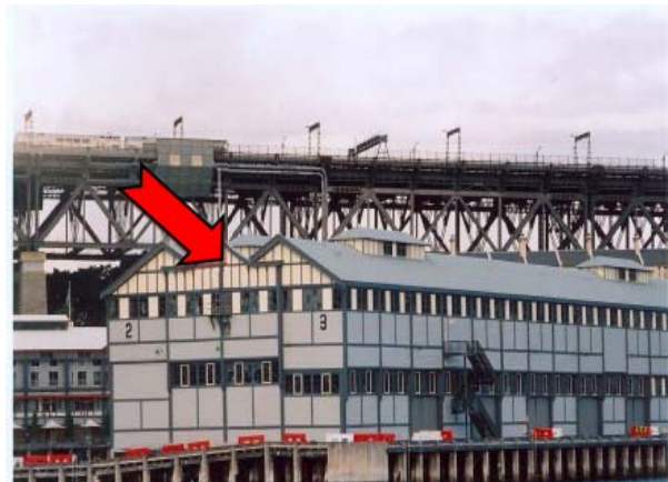
Photo 4. Exterior/interior, level 1, north wall, gable infill panel – suspected asbestos-containing fibre cement sheeting
