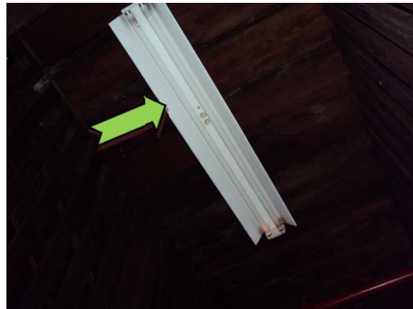
Photo 10. Interior, ground level, central, northern stairwell, ceiling throughout, double tube fluorescent light fittings – suspected negative for the presence of PCB-containing capacitors
