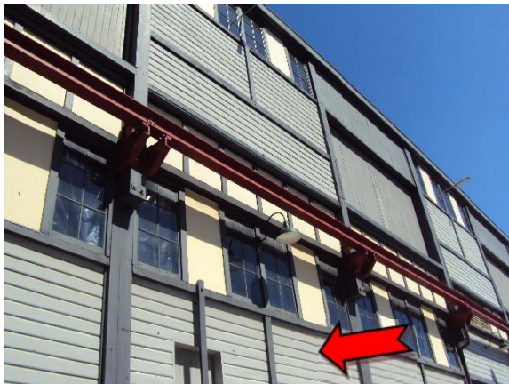
Photo 11. Exterior, throughout, timber features – lead-containing white lower colour paint system
