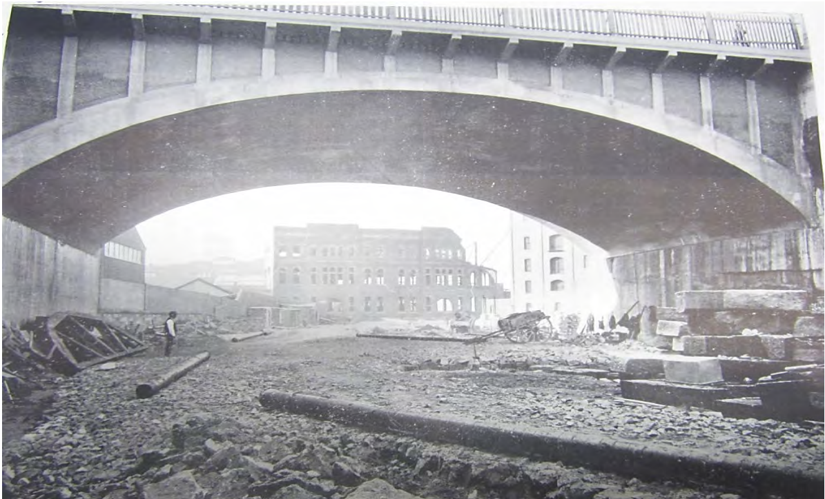
View west along Hickson Road showing the new bridge that spanned what was described as “deep rock cutting” through Millers Point. Wharf 8/9 is in the background and in the foreground can be seen some of the sandstone that has been extracted as dimension stone (Source: SHT Annual Report 1913)
