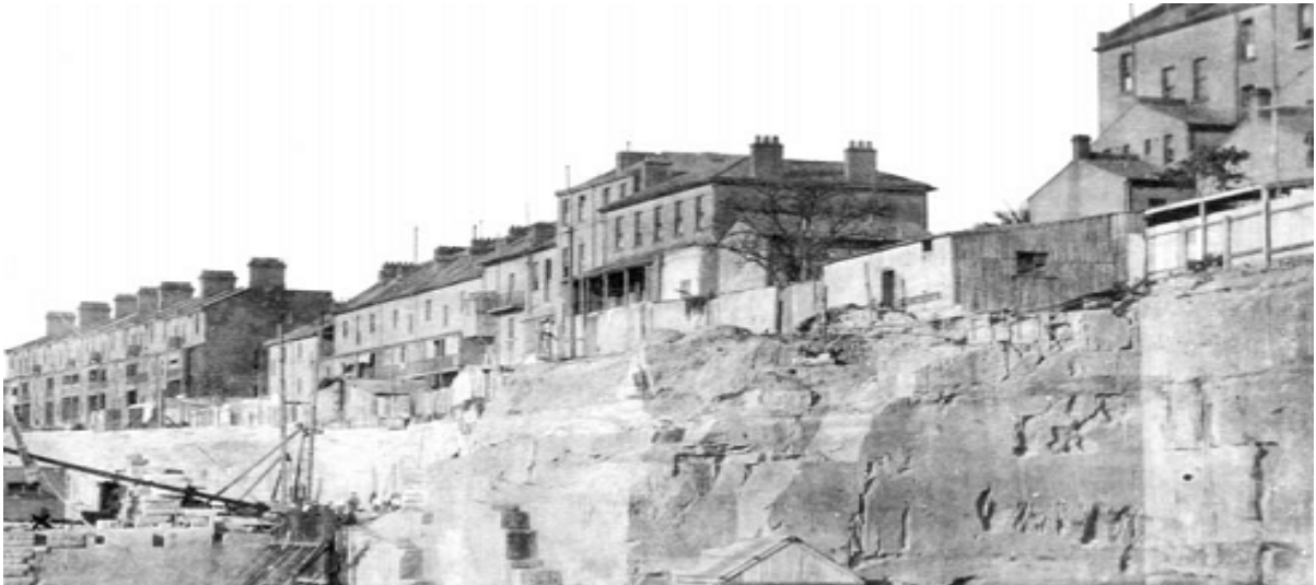
The extent of excavation of the existing landform required to create the new streets of Hickson Road and New Pottinger Street is demonstrated in this image (Source: GPO collection reproduced in Fitzgerald and Keating (1991), Millers Point the Urban Village )
