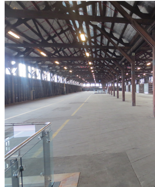
Figure 28: Upper Shed, roof structure and trusses, Pier 2/3
