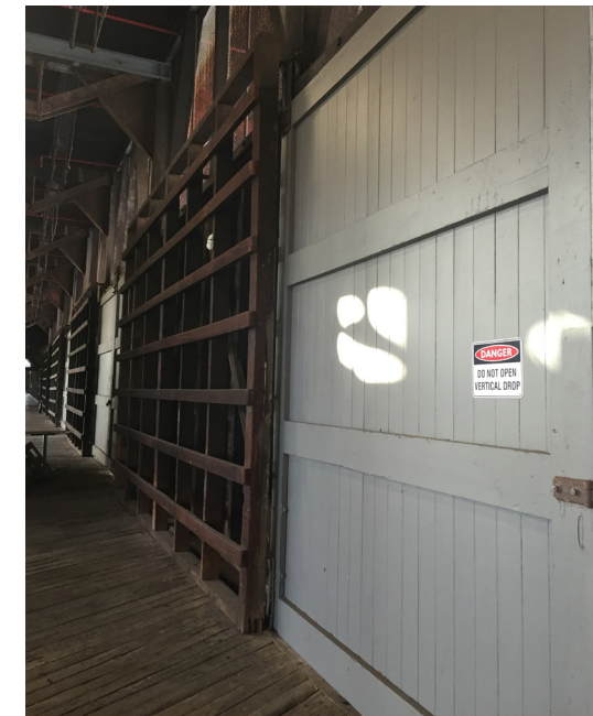
Figure 26: Existing timber door protectors and painted timber cargo doors, Pier 2/3
