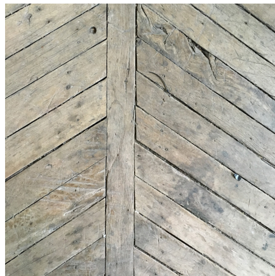
Figure 40: XTF Existing timber floor, repaired.
