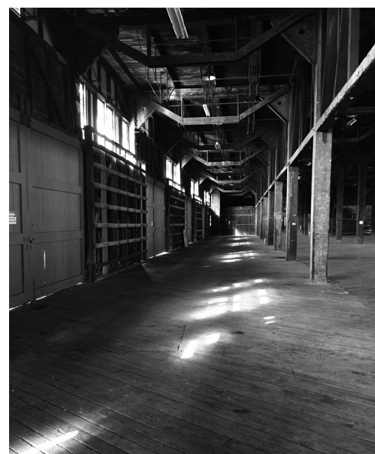
Figure 30: Lower Shed, Pier 2/3
