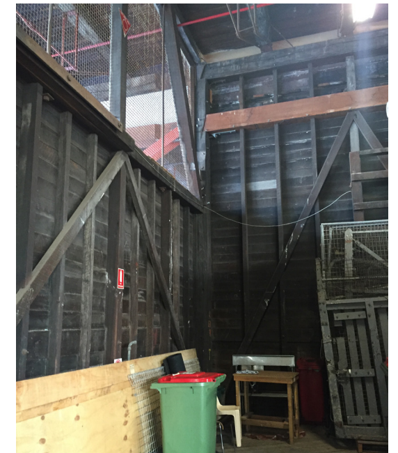
Figure 27: Existing timber wall cladding and structure, Pier 2/3
