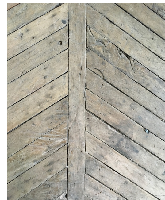
Figure 25: Existing timber floor, ground floor, Pier 2/3 The upper shed timber floor is currently covered in bitumen.
