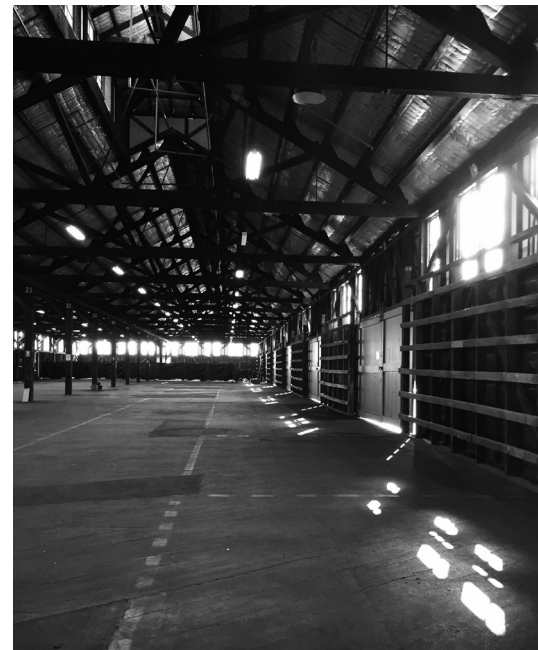
Figure 29: Upper Shed, Pier 2/3
