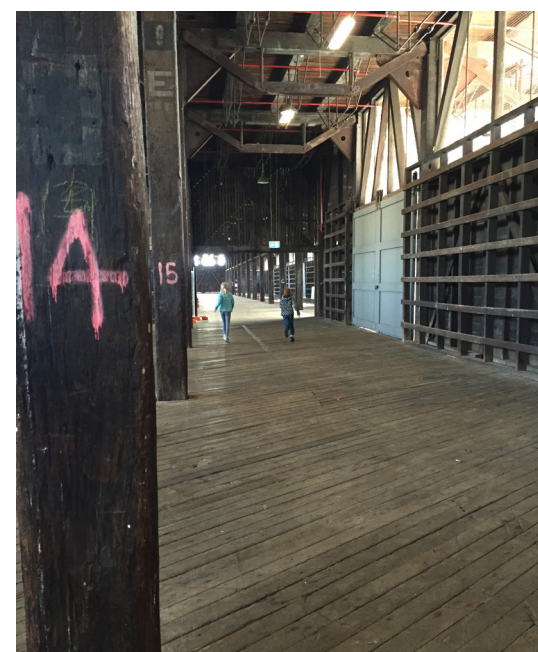
Figure 31: Lower Shed, Pier 2/3
