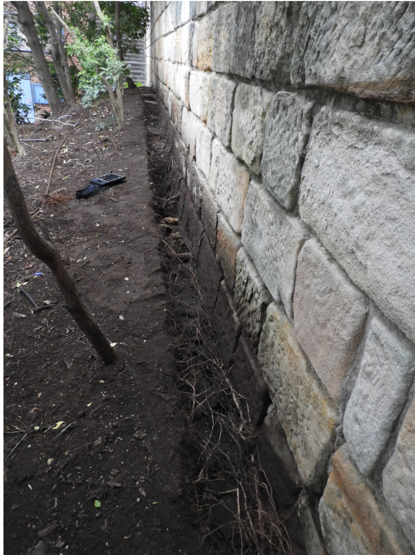
Figure 1. An image of the excavated trench along the base of the sandstone retaining/boundary wall. Source: ArborSafe, October 2018
