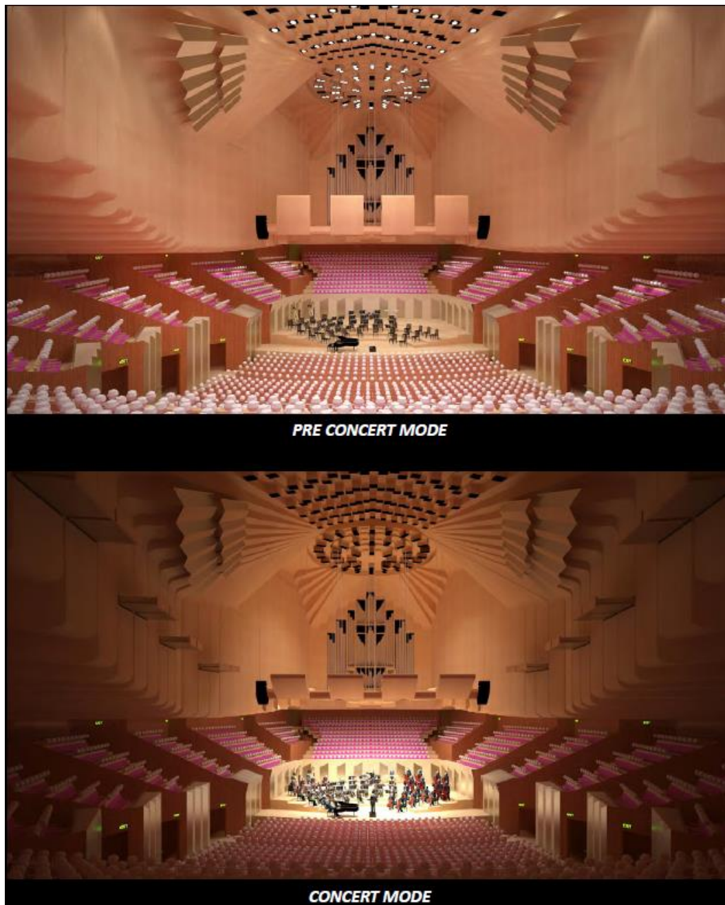
Figure 40: Concert Hall Concept Design – Acoustic Reflectors shown in Pre-Concert and Concert Modes
