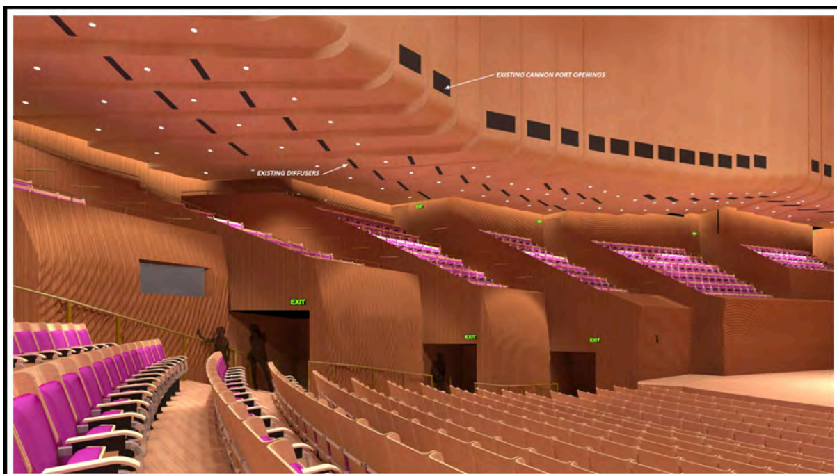
EXISTING SLOT DIFFUSERS & CANNON PORT OPENINGS
