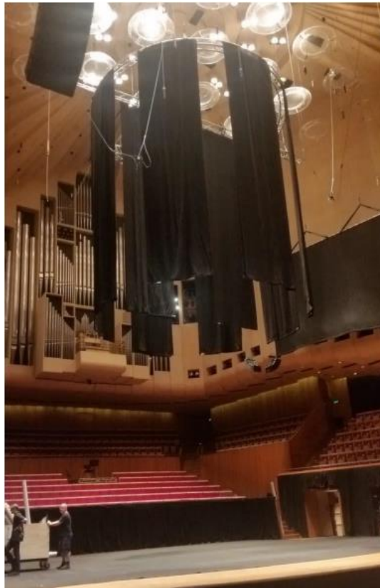
Figure 16: Absorbing curtains around the stage, absorbent carpet on stage (setup not finished)
