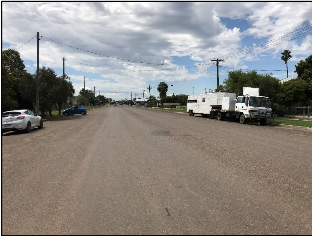
Photo 8 – Typical cross section along Bloomfield Street allowing for kerb side parking and two-way heavy vehicle movements
