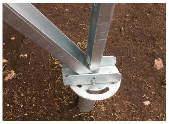
Figure 3-6 Example of ground mounting arrangements
