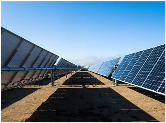
Figure 3-7 Example of Tracking Solar PV panels
