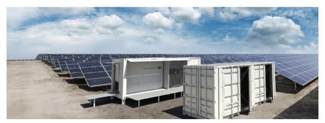
Figure 3-9 Example inverter station
