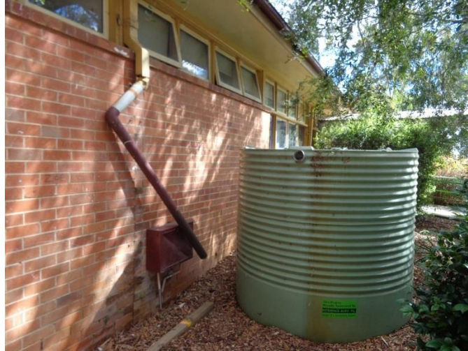
Existing Rainwater Reuse Tank
