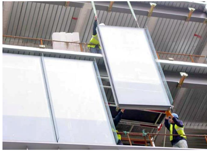
Figure 34: Example of curtain wall panel installation
