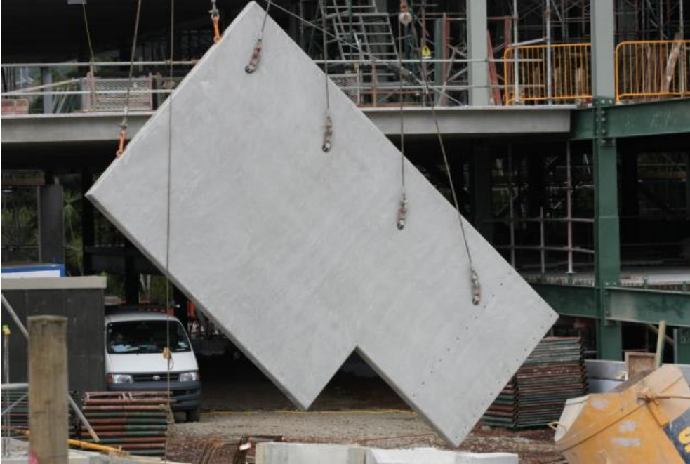
Figure 28). Panels will be lifted by crane to their final positions.
