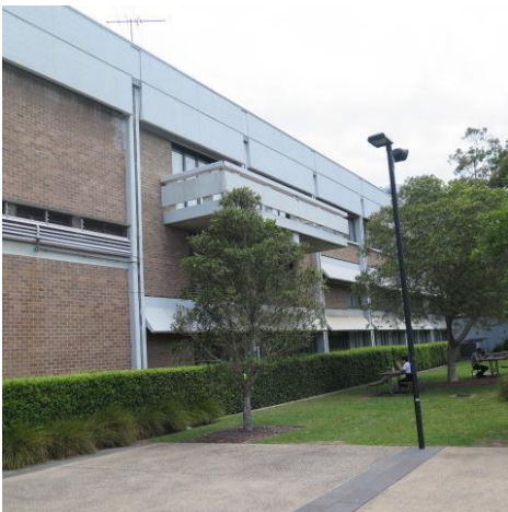
Figure 17 – North Elevation of Electrical Engineering building showing the off-form concrete structure (with later addition paintwork) and infill face brickwork. The podium to the northern wing (in foreground) comprises two levels. The southern wing is a seven level tower. Sun louvres and awnings are located over window openings.
