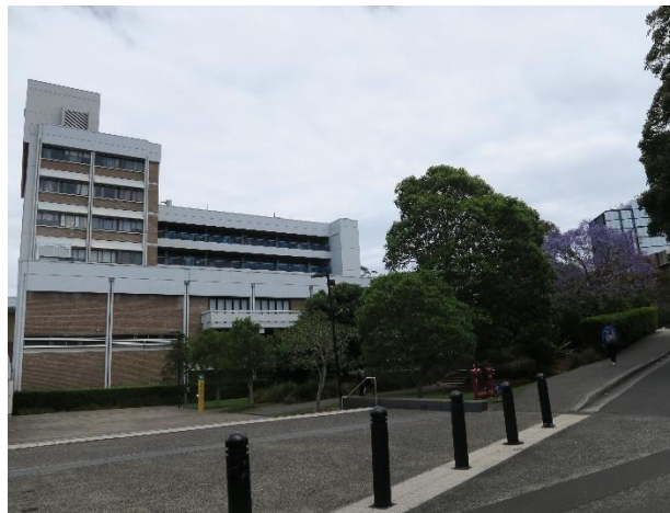
Figure 17 – North Elevation of Electrical Engineering building showing the off-form concrete structure (with later addition paintwork) and infill face brickwork. The podium to the northern wing (in foreground) comprises two levels. The southern wing is a seven level tower. Sun louvres and awnings are located over window openings.
