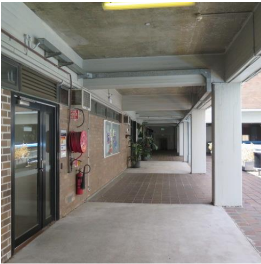
Figure 16 – View looking east along the internal balconies to Electrical Engineering building. Materials include off-form concrete structural system (columns, beams and slabs) with infill brickwork walls and metal framed window and door openings. Paint to the concrete is a later addition. Floor has quarry tile and concrete finish.
