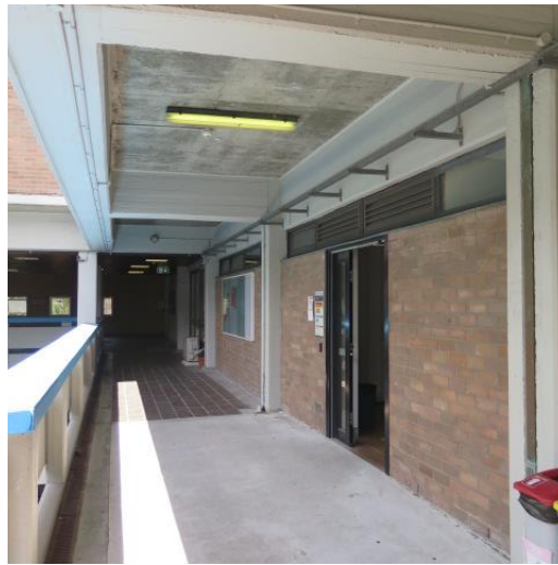
Figure 16 – View looking east along the internal balconies to Electrical Engineering building. Materials include off-form concrete structural system (columns, beams and slabs) with infill brickwork walls and metal framed window and door openings. Paint to the concrete is a later addition. Floor has quarry tile and concrete finish.
