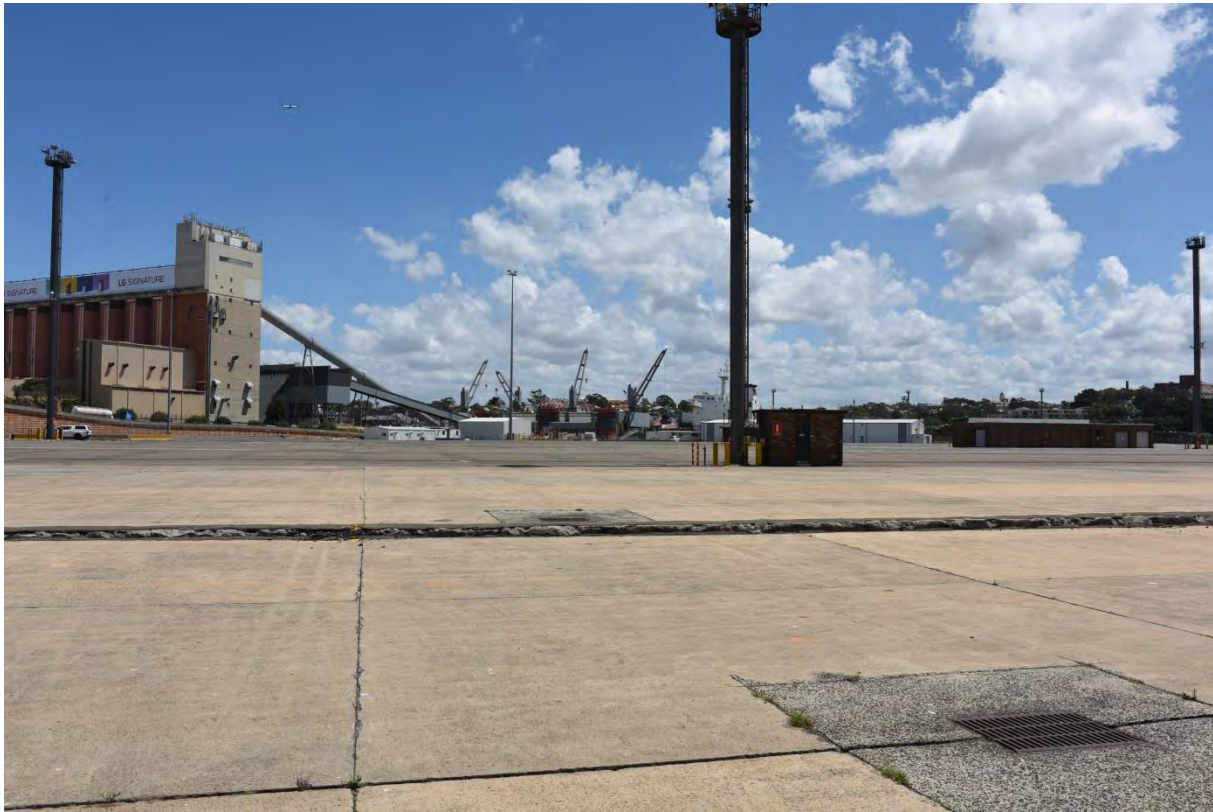
Figure 10 Stormwater on Glebe Island is collected in local stormwater pits scattered across the wharf and hardstand area (Source: AECOM)
