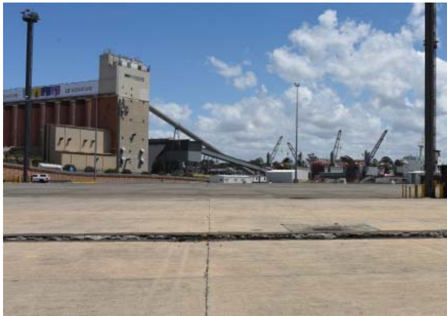
Figure 7- View facing north west of the Site towards the cement processing plant (west) and the White Bay locality further beyond
