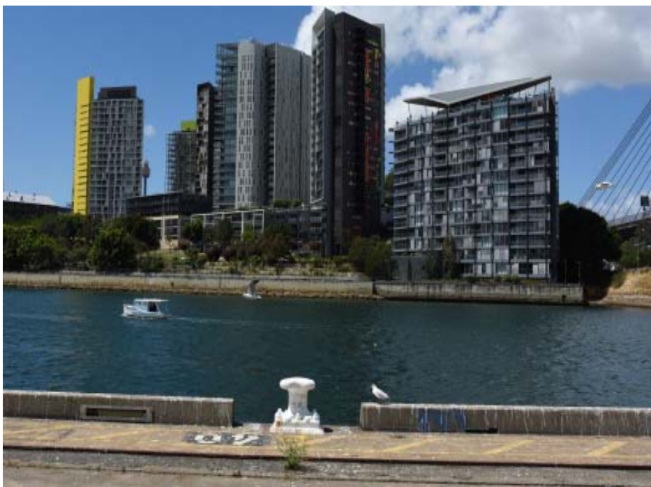
Figure 9- View of Pyrmont Waterfront Park and Pyrmont Peninsula across Jones Bay east of the Site
