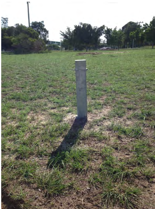
PHOTOGRAPH 10 Existing intact monitoring well located in north-west corner of site
