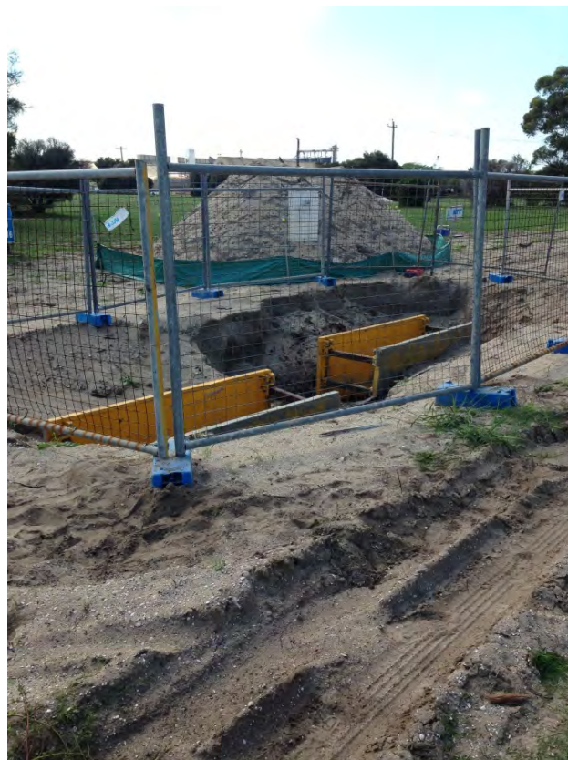
PHOTOGRAPH 12 Construction work in south-east corner
