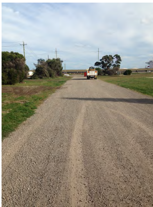
PHOTOGRAPH 2 Looking south from north-east corner, showing access road on eastern side of site
