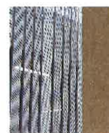
6 - LOUVRES - CAR PARK
