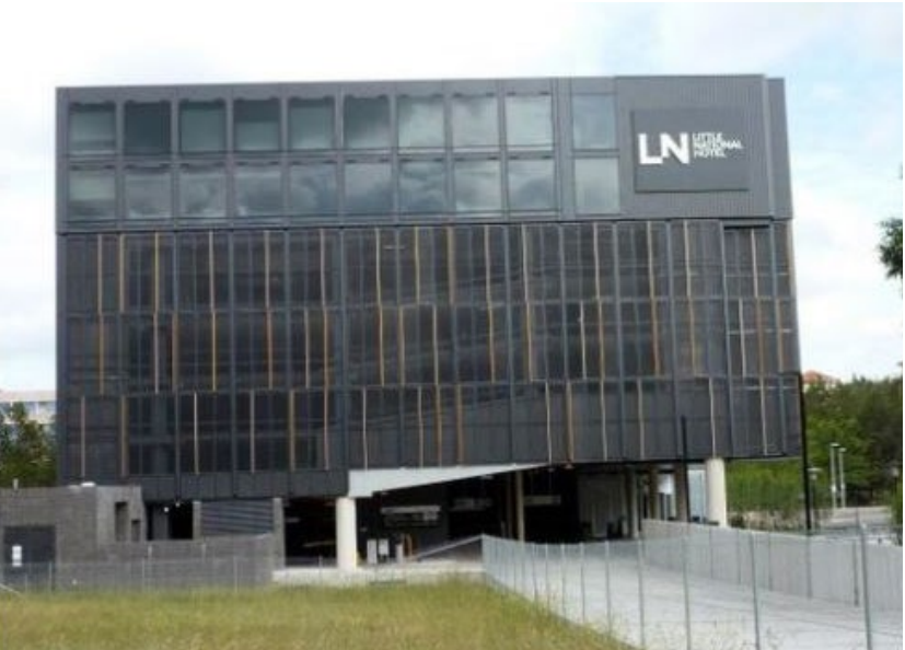
Above is an example of the same typology which uses mechanical ventilated rooms and large inoperable fixed windows.
