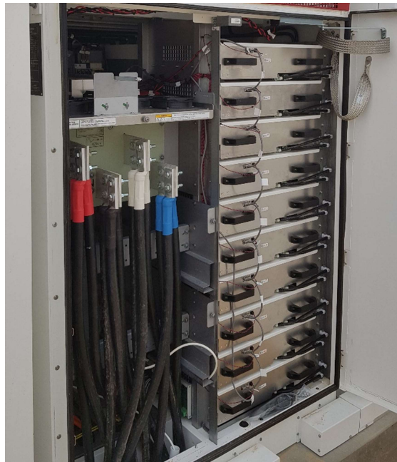
Figure 3.1 - battery cubicle showing field replaceable pods
