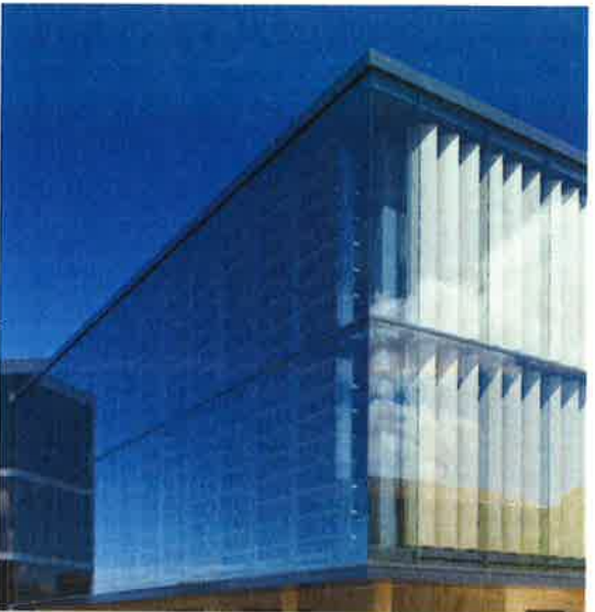
Glazed twin wall facade with integral aluminium sun shade louvers
