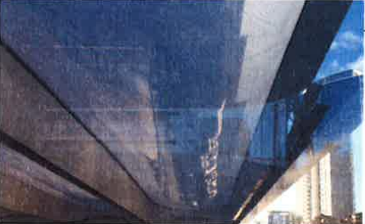
ETFE roof - view from below
