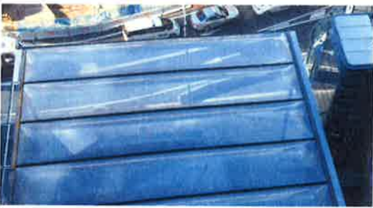
ETFE roof - view from above
