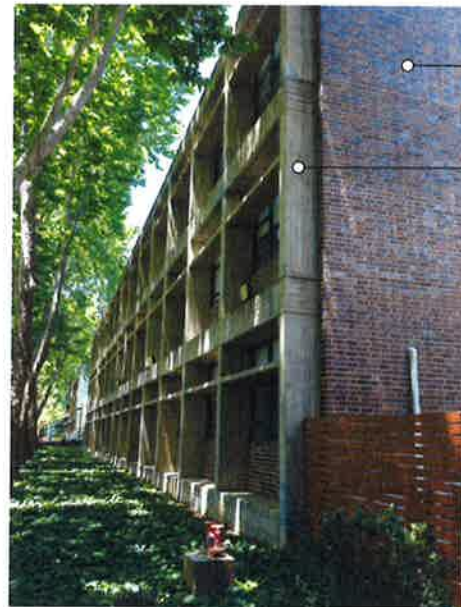
Existing site photo- 25WWA north facade
