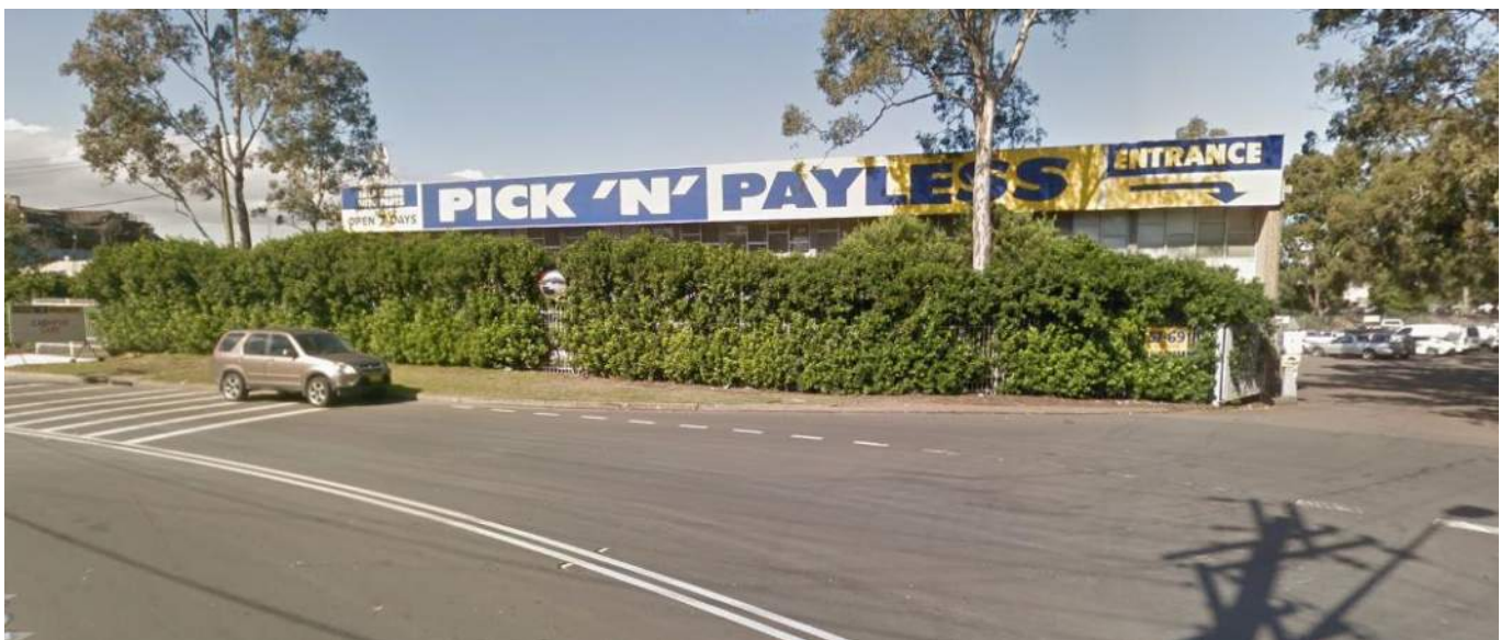
Photograph 3: View of the Subject Site from Tattersall Road - Looking South. Western driveway entrance on the far right.
