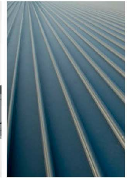
Metal deck roofing
