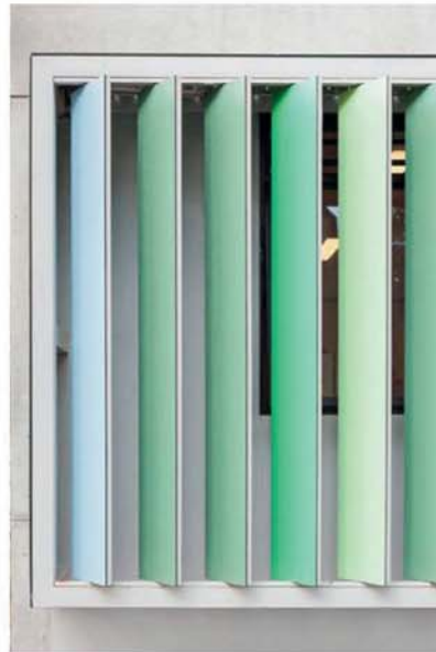
Powdercoated vertical louvres to south, east and west facing homebases
