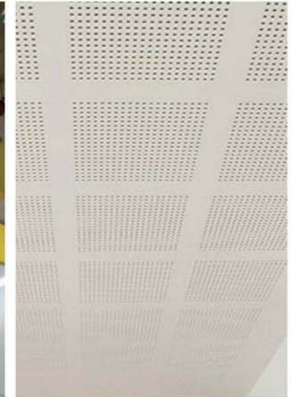
Perforated plasterboard ceiling to homebases, group rooms and hall
