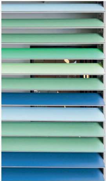
Powdercoated horizontal louvres to north facing homebases
