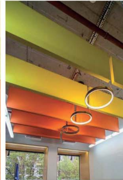
Baffle ceiling to maker spaces and library
