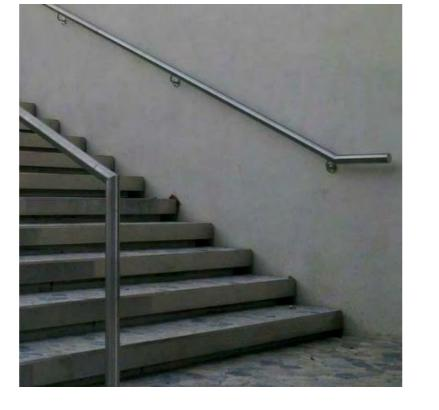
BAH-01 SS Handrail Architectural Metalwork Stainless steel tubular handrail to locations nominated on the Design
