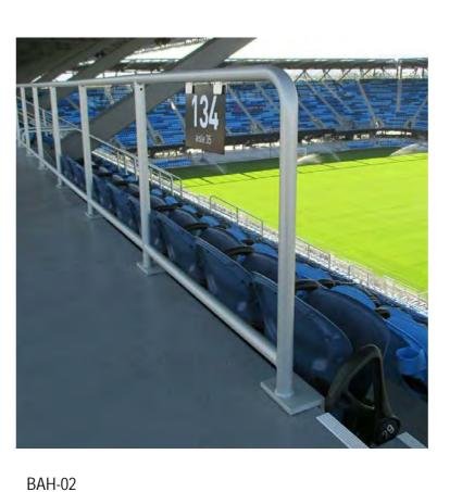
Galv Steel Handrail Architectural Metalwork
