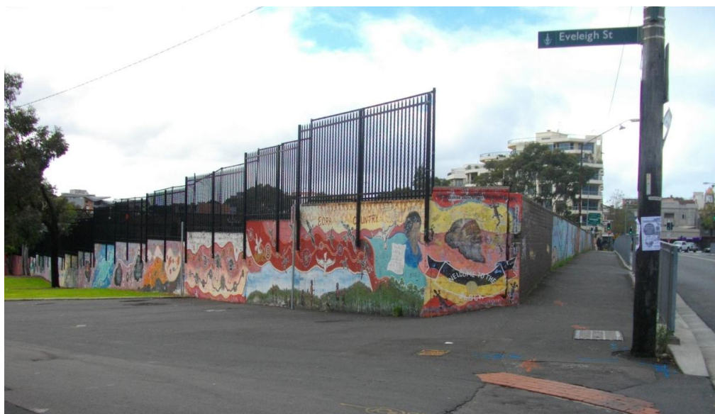
Figure 22 – View from the corner of Eveleigh and Lawson Streets looking north northeast of the boundary walls showing the mural painted stepped concrete block wall to the left and the railway bridge wall to the right (Source: NBRS+PARTNERS, June 2011)
