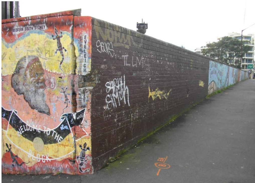
Figure 26 – View of the corner, showing the junction of the English bond brick wall to Lawson Street (right) and the mural painted concrete block wall to Eveleigh Street (left) (Source: NBRSPARTNERS, June 2011)
