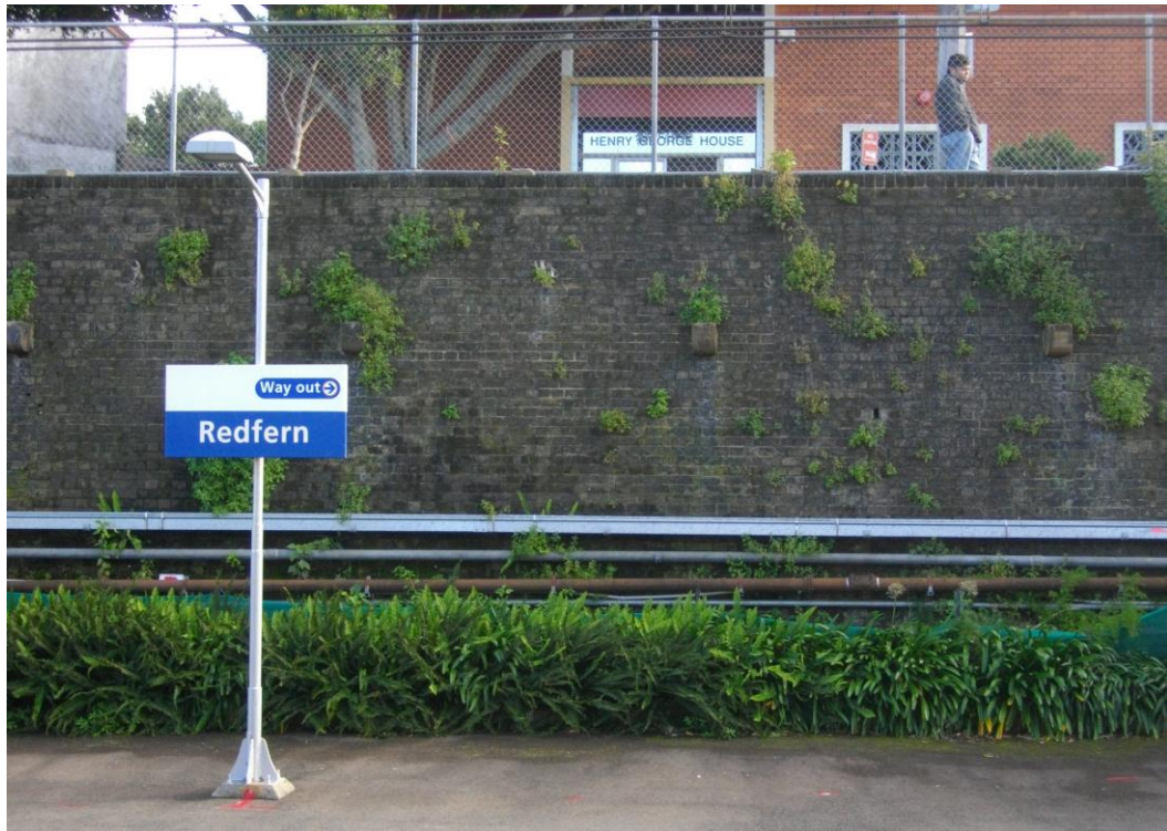
Figure 21 – View north to the brick retaining wall along Platform 1 at Redfern Railway Station. This retaining wall appears to be the same construction as the railway corridor on the retaining wall to the north (Source: NBRS+PARTNERS, July 2011)
