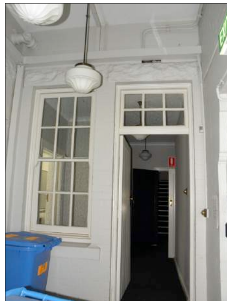
Figure 37: Doors between Rooms G02 and G03. Neither door is original. It is proposed to remove the timber framed and glazed door.
