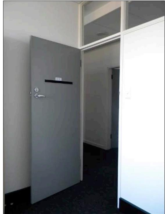
Figure 108: Typical door in the north-south wing. Also showing a detail of the partition wall with fixed fanlights that line both sides of the corridor. This wall at this level is masonry.
