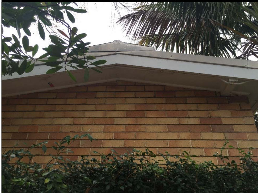
PHOTOGRAPH 16: SUSPECTED ASBESTOS EVES
