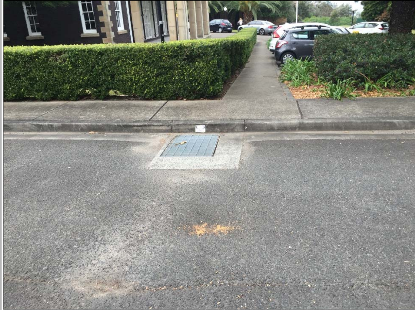
PHOTOGRAPH 11 – STORMWATER SYSTEM PRESENT WITHIN THE WESTERN CARPARK
