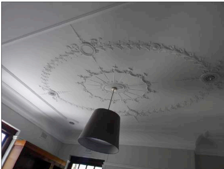
Figure 2: Interwar period plaster ceiling and cove cornice.
