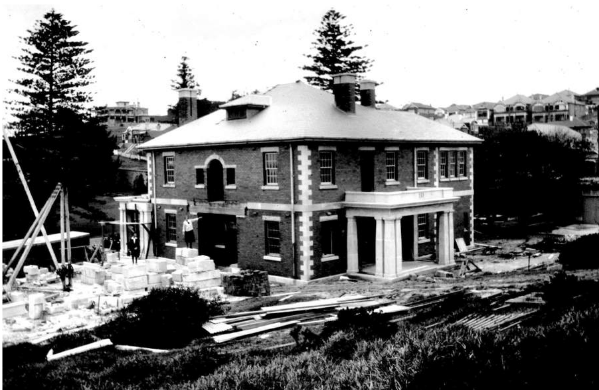
Figure 36: Cliffbrook under Construction - Stone terrace and portico construction in progress (c.1921/22)
