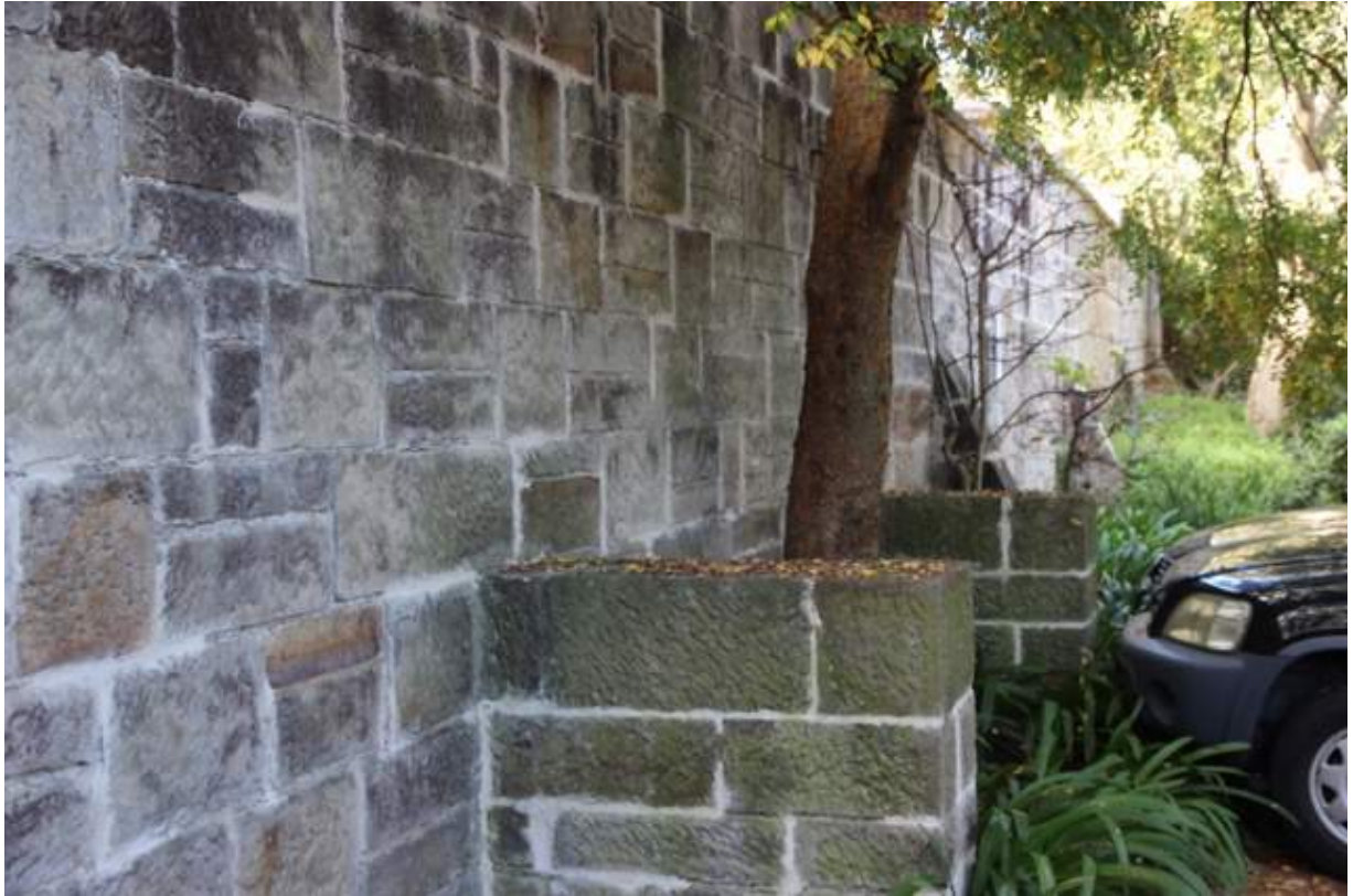
Figure 57: Cliffbrook Campus (northern boundary wall buttressing)
