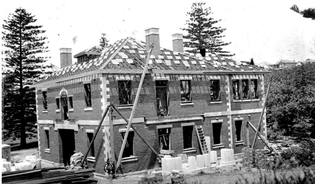
Figure 34: Cliffbrook under Construction - Slate roof works & stone detailing in progress (c.1921/22)
