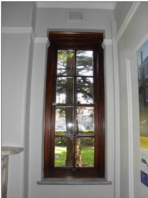
Figure 4: Detail of the window in the western wall, showing the white marble sill common to windows at this level.
