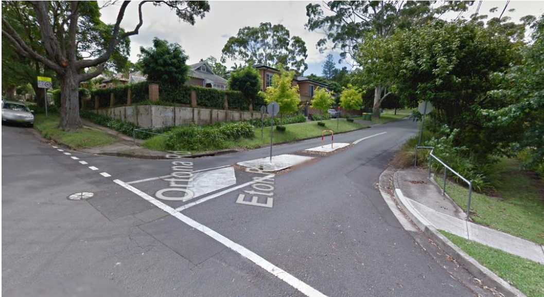
Photo 3: Improper splitter island at Eton Road / Ortona Road intersection (Google Street view 2016)
