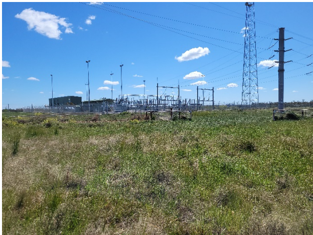
Plate 5-6 Electricity easement, powerplant, fences
