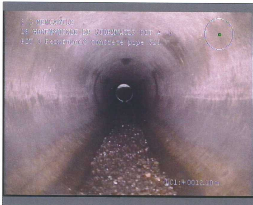
Photo: 3_3A 12.1m, Ingress of soil, fine material , at 6 o'clock, Start
