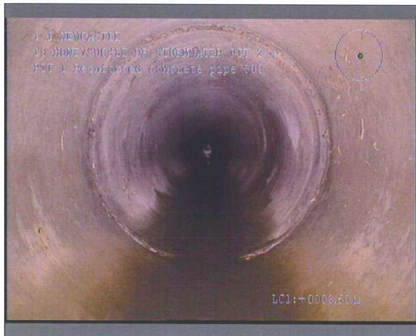
Photo: 1_3B 3.6m, Joint displaced longitudinally, longitudinal displacement 10-20mm
