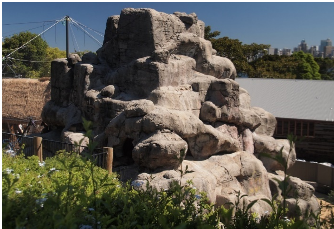
Figure 70 A 2017 view of the 1932 Tahr Mountain, though now showing within its traditional setting visually intrusive structures associated with the new Sumatran Tiger precinct to the south. Also note the current 'blocky' form of the structure after modifications to its original 'angular' form ( Figure 11 ) – ostensibly to assist with regular cleaning and maintenance though, in practice, this has not been convincingly successful. (Courtesy: Geoff Ashley)
