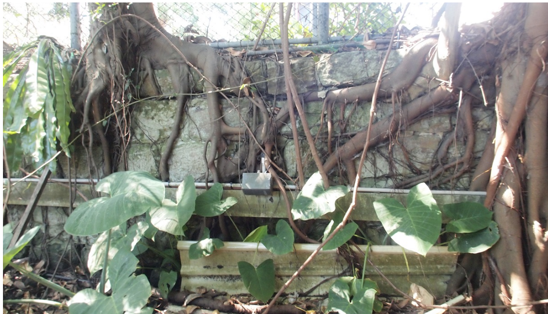
Figure 111 Between the former Finch Aviaries and the large fig tree (Item 160L) is a meandering retaining wall of mixed construction though mainly sandstone ashlar blockwork along the western half. It is presently enshrouded in a combination of fig tree seedlings, foliage and sundry services.
