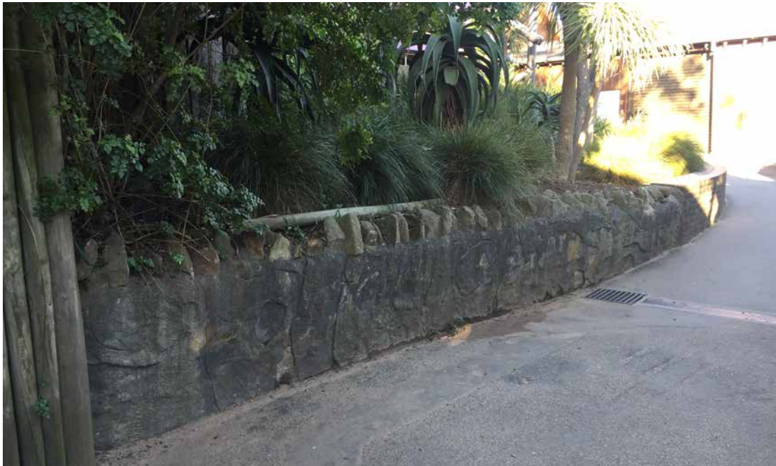
Figure 97 Item I32L, near the eastern end of the Waterhole precinct, features faux-rockwork render to the body of the wall with stone cresting reminiscent of that used for the one-off rustic stone exedra and bridge within the eastern gully of the zoo. Its character and position defining an early path, suggest the wall section was part of the early phase of zoo development.
