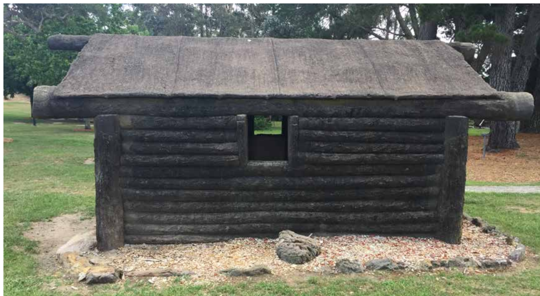
Figure 69 The concrete faux-timber log shelter at Mount Victoria in the Blue Mountains also showing its parallel-scored roof cladding to imitate traditional thatch. Both this structure and the 1940s giraffe house at Taronga Zoo share in common the technical expertise and creative authorship of Tom Adam.
