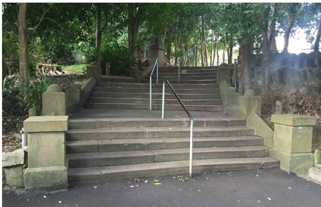
Figure 110 Ensemble of curving sandstone steps and associated detailing. Note the internal piers with balled surmounts as a contrast to the plainer, principal piers with flat coping suggesting the intended addition of features as part of the original design.
