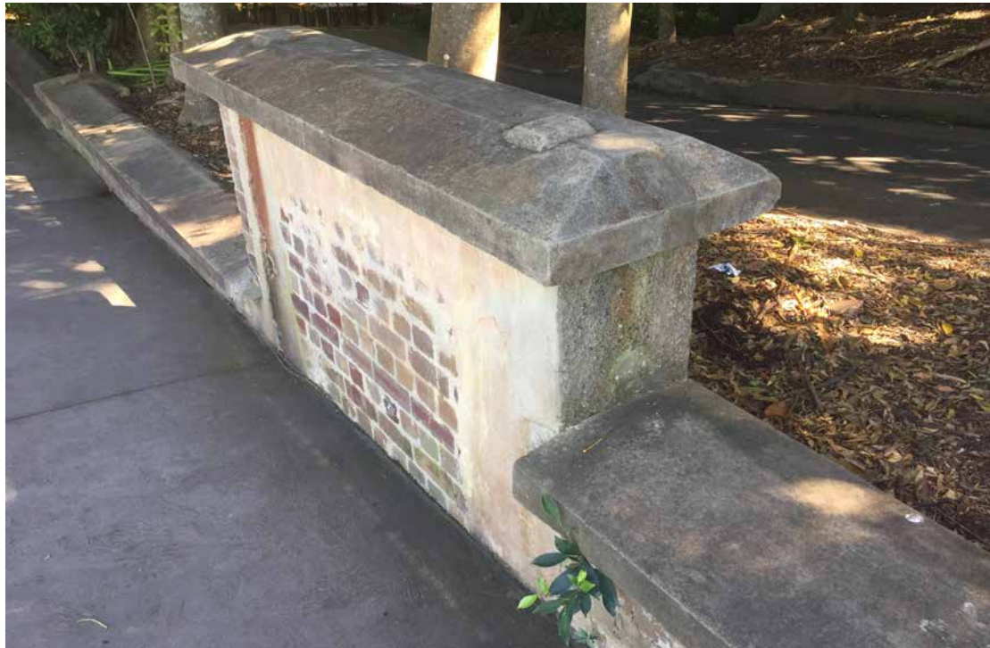
ABOVE Figure 84 Part of the upper boundary wall of the former Birds of Prey aviary showing its generous concrete coping and an upstand section with exposed English Bond brickwork. BELOW LEFT Figure 85 An intact corner section of the former aviary boundary wall. BELOW RIGHT Figure 86 Callitris rhomboidea at the end of the former Birds of Prey aviary – and potentially contemporary with it.
