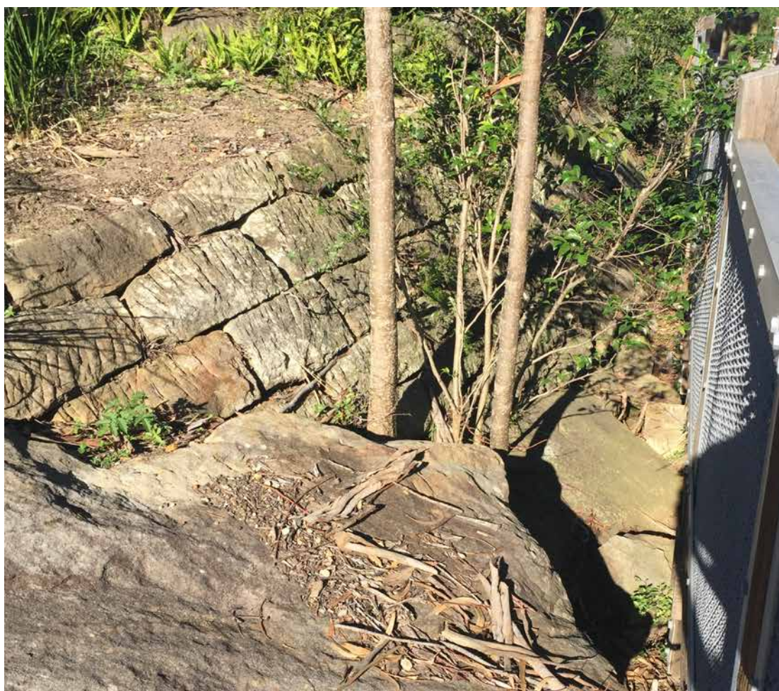
Figure 96 A section of battered drystone retaining wall of worked (sparrowpecked) sandstone above the existing ramp (at right) and south of the Barbary sheep enclosure. Note too, part of a large rock outcrop in the foreground that characterises the remnant natural landscape in this western part of the Waterhole precinct.
