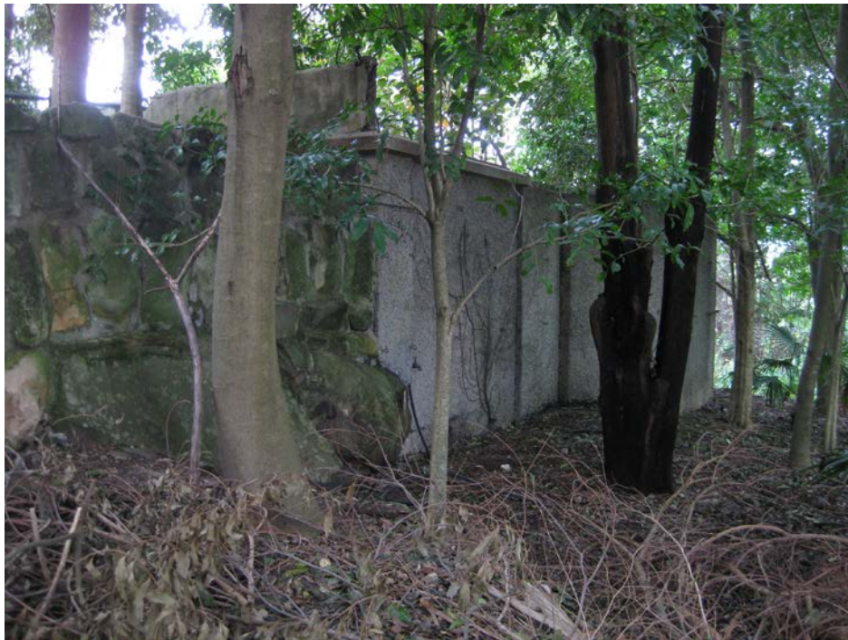
Photo 7 – Retaining wall founded on rock
