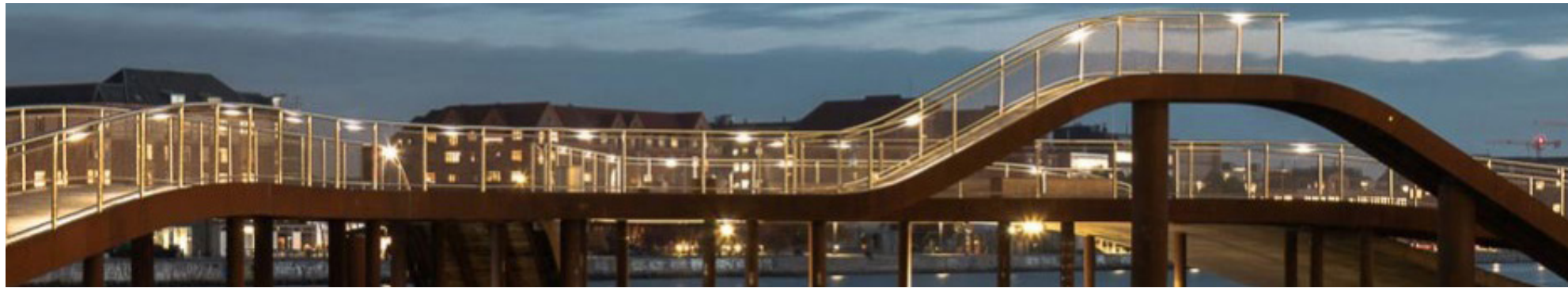
Kalvebod Waves, Copenhagen Denmark
