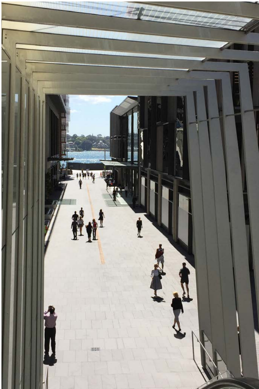
3. VIEW FROM NAPOLEAN BRIDGE - STAGE 1A
