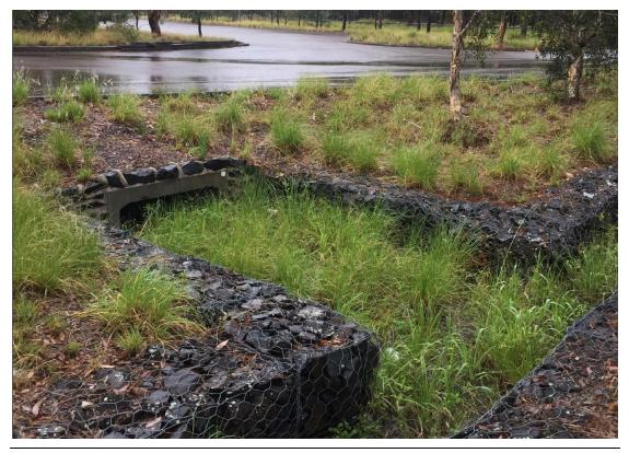
Figure 8: Typical existing vegetated swale
