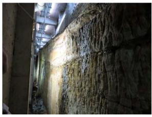
Figure 3.30 The Services corridor that runs along the southwest side of the building. The degree of excavation of sandstone that was required to construct the building is evident. (Source: GML, November 2016)
