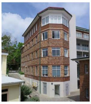
Figure 3.14 The Marian Centre, as viewed from the east. The top floor later addition can be seen. The lift shaft (later addition) is rendered and painted grey. (Source: GML, November 2016)
