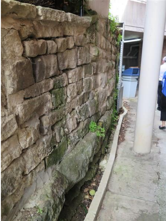
Figure 3.5 Retaining wall between the Marian Centre and B-Block. The natural sandstone bedrock is visible at the bottom of the retaining wall. (Source: GML, 2016)
