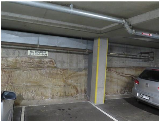
Figure 3.11 Underground carpark. Excavation into the bedrock. (Source: GML, 2016)
