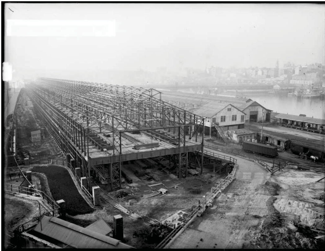
FIGURE 14: FRAME WORK OF DARLING HARBOUR SHEDS CONSTRUCTION, NEW SOUTH WALES (C1920). IMAGE SHOWS THE 1902 OUTWARDS GOODS SHED A&B AT THE RIGHT, THE 1891 SHED C&D IN THE CENTRE AND THE 1823 DOUBLE TIER SHED AT THE LEFT UNDER CONSTRUCTION. SOURCE: NLA PIC P860/325 LOC COLD STORE PIC AGF
