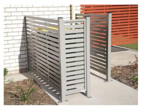
Figure 3 Example of waste bin screening – slat fencing colourbond (or similar)
