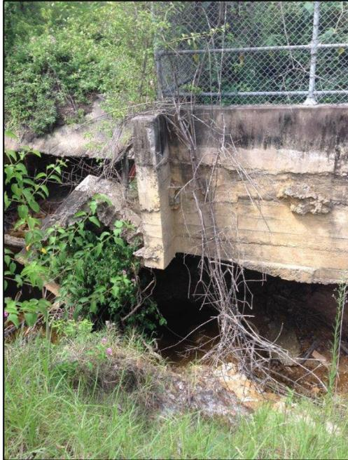
Photo 5-4: Channel failure and scouring westward scouring
