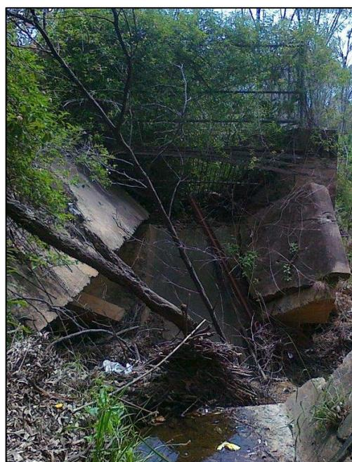
Photo 5-3: Channel failure and scouring viewing downstream (westward)
