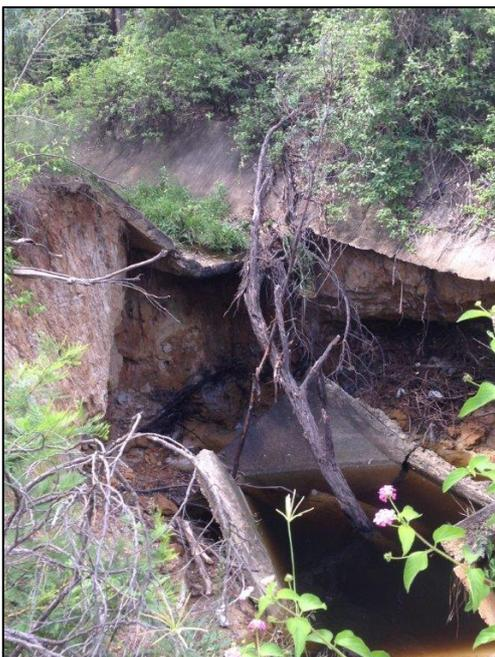
Photo 5-2: Channel failure and scouring viewing upstream (eastward)
