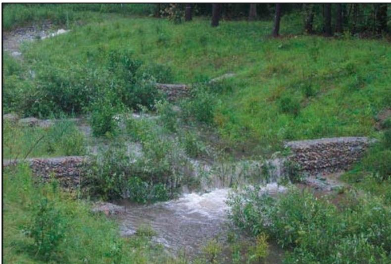
Photo 5-6: Vegetated gabion structures
