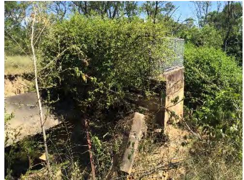
Vegetation downslope of existing drain in basin 5 Outlet Existing damaged/collapsed drainage structure
