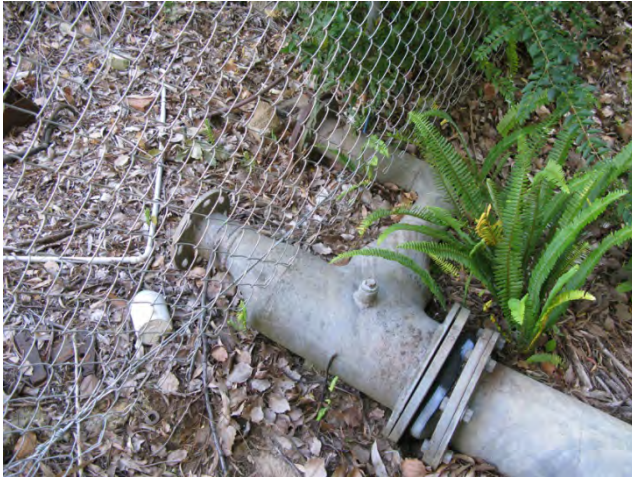
Fig A.4 Amiens wetland 25/05/2016 Disconnected pipe at south western tip of wetland, purpose unknown
