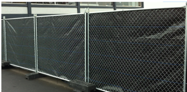
Figure 9. Example temporary fence
