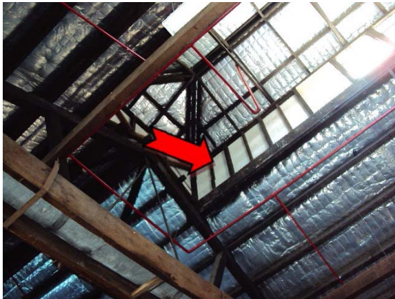
Photo 1. Exterior/interior, upper roof gables (north and south), infill panels – suspected asbestos-containing fibre cement sheet
