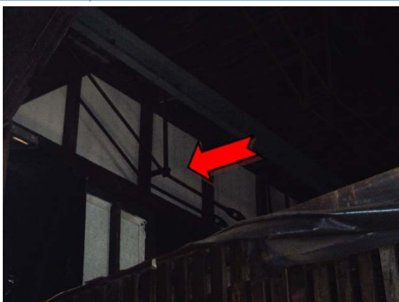
Photo 5. Interior, ground level, throughout, infill panels to windows – suspected asbestos-containing fibre cement sheeting
