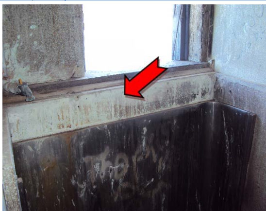
Photo 6. Interior, level 1, north toilet, infill panels to urinal and windows – asbestos-containing fibre cement sheeting
