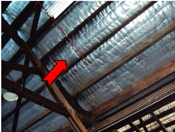
Photo 7. Interior, level 1, ceiling throughout, sarking – suspected SMF-containing insulation material
